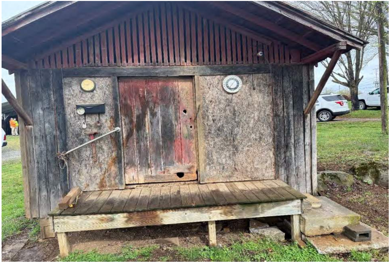
11 Subject Property - Grain Shed - Facing W.jpeg
