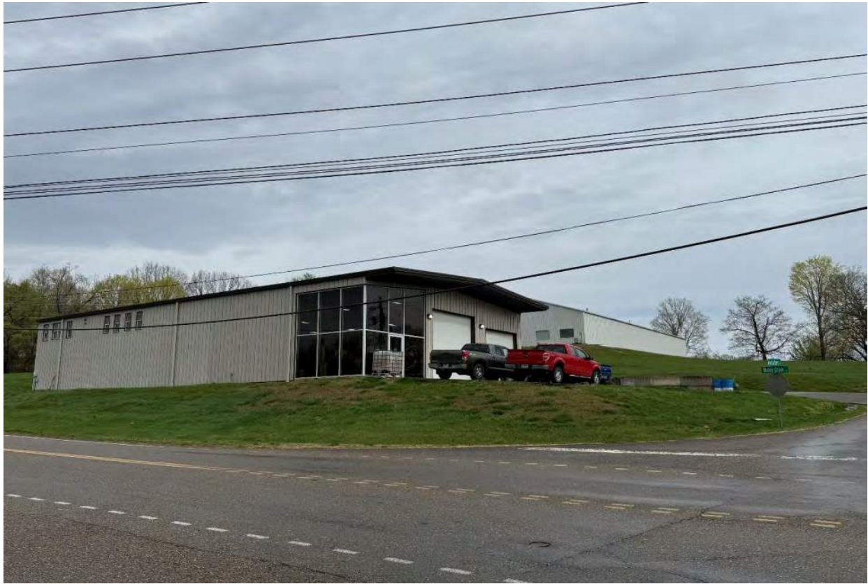
19 RMI Machine Shop - Facing N.jpeg
