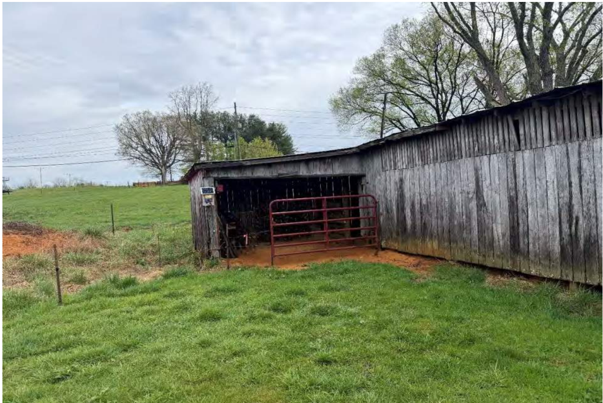
10 Subject Property - Equipment Shed - Facing N.jpeg
