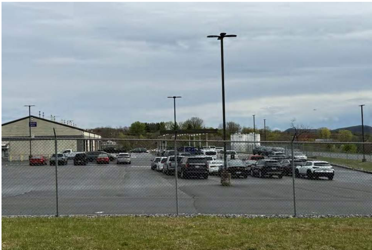
18 Tri-Cities Airport Fueling Facility - Facing N.jpeg
