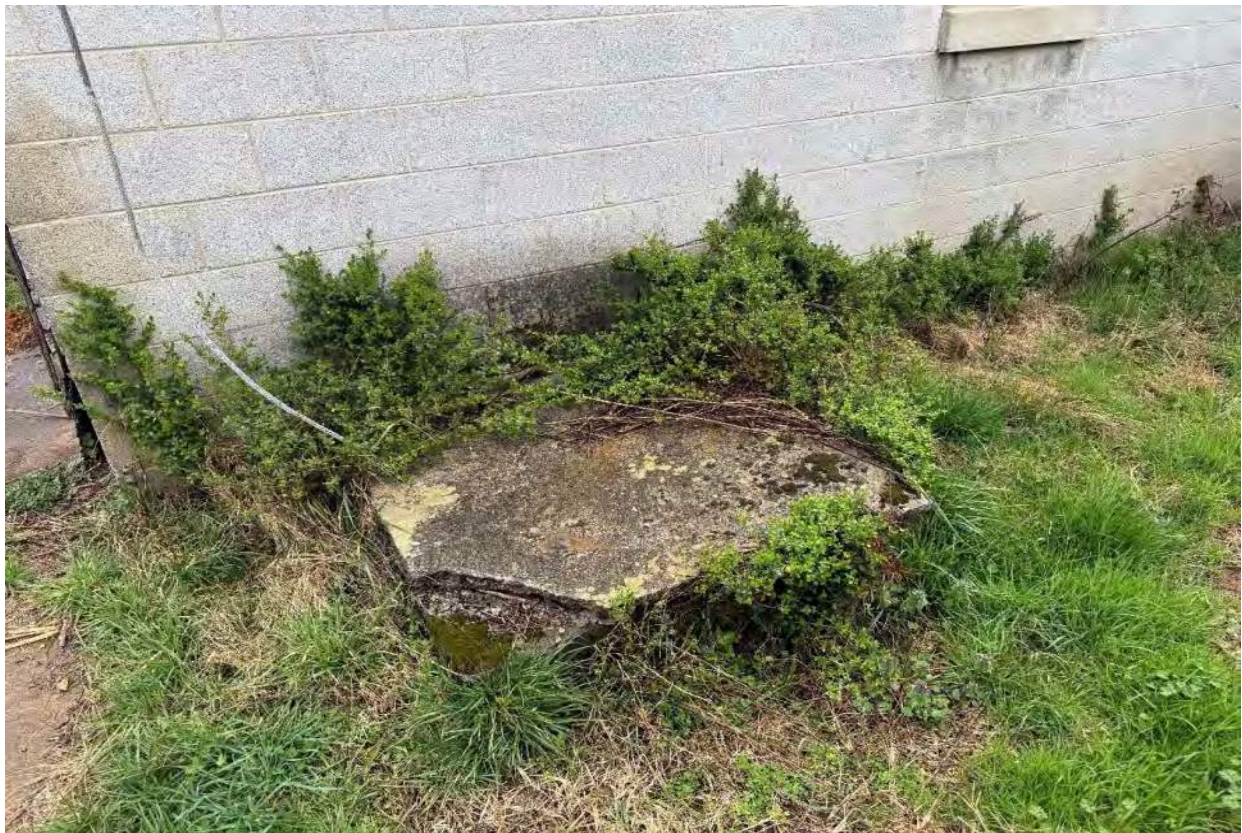
14 Subject Property - Cattle Waste Cistern - Facing N.jpeg
