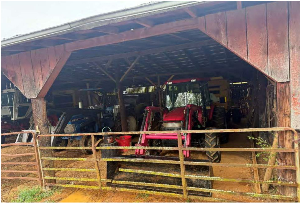
09 Subject Property - Equipment Shed - Facing W.jpeg
